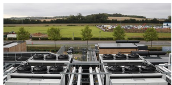
Installation of a sophisticated system of partially solar powered heat pumps to heat and cool the Cambridge Movement Surgical Hub.
